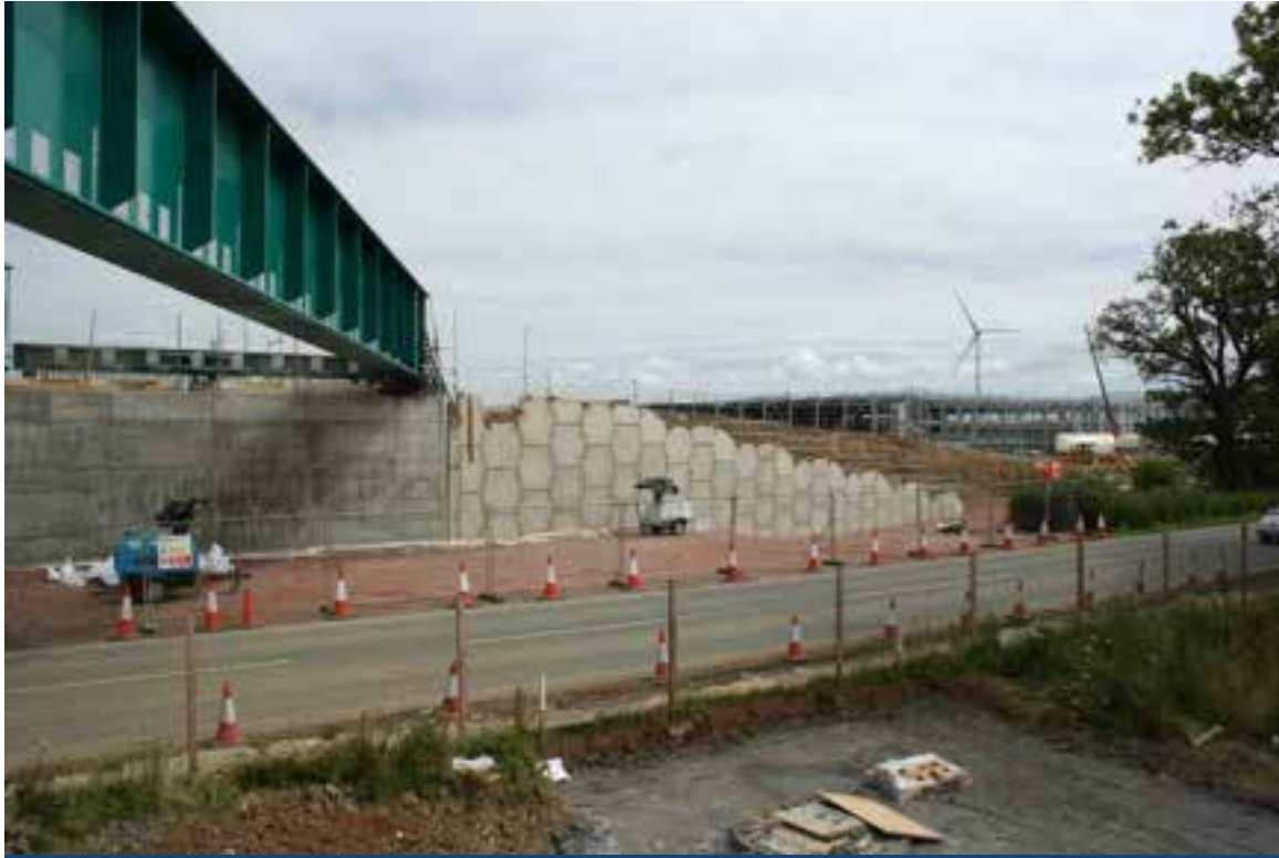
Concrete Panel Reinforced Earth Wing Wall with new warehouse in background
