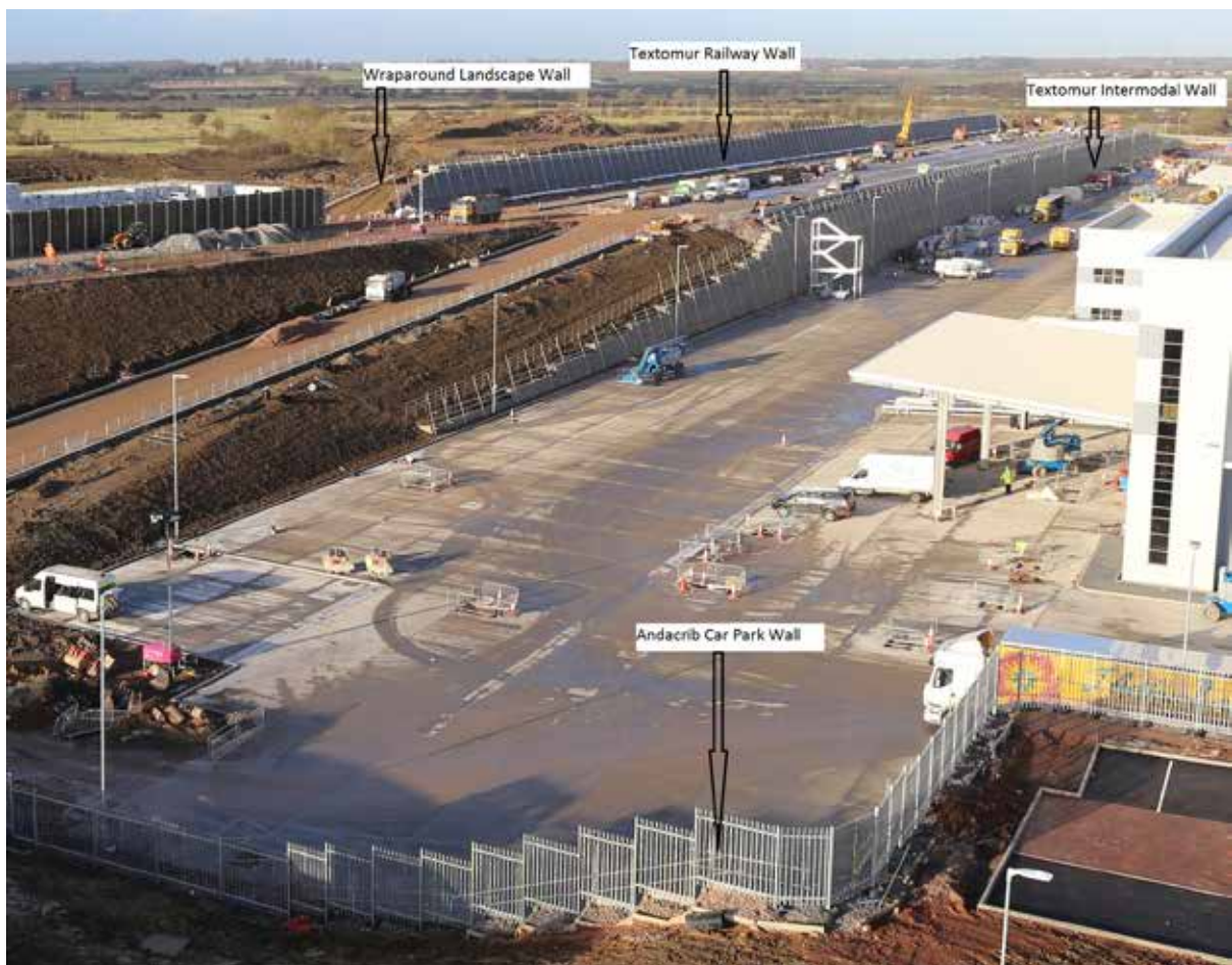
Completed Structure. Taken October 2014
