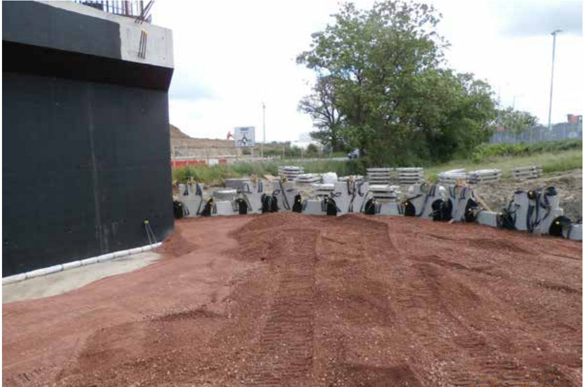
Concrete panels with polymer strap reinforcement ready to be laid out
