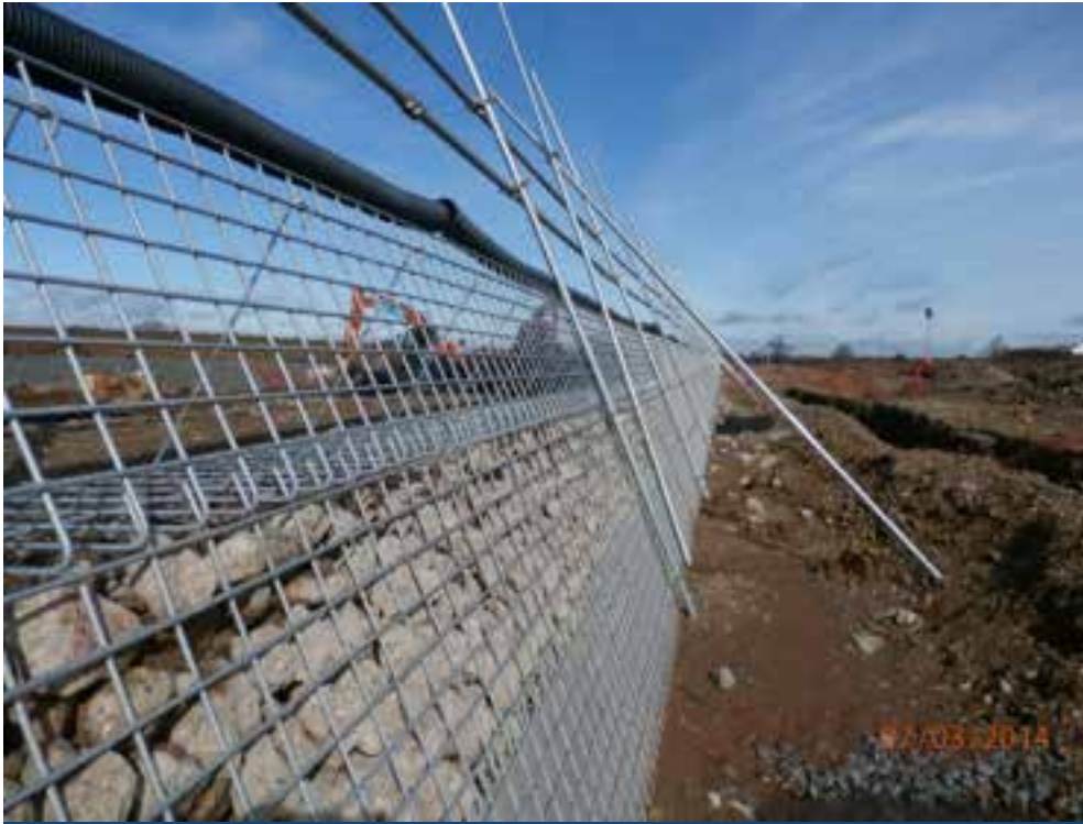
Galvanised Textomur cages prior to filling with recycled crushed concrete.
