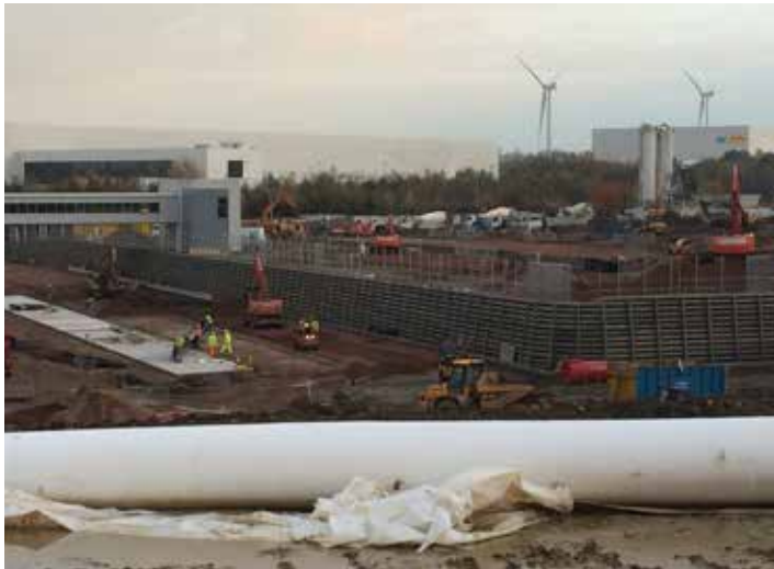
Andacrib Concrete crib retaining wall supporting the new car park.
