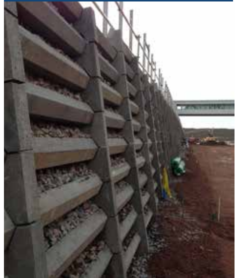
Andacrib Concrete Crib Wall
